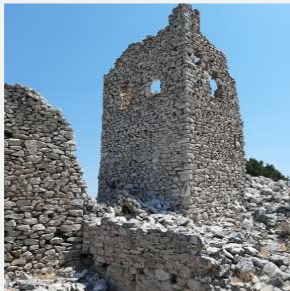
Image 3 Rizokastro Aliveri, view of the tower inside the castle.
